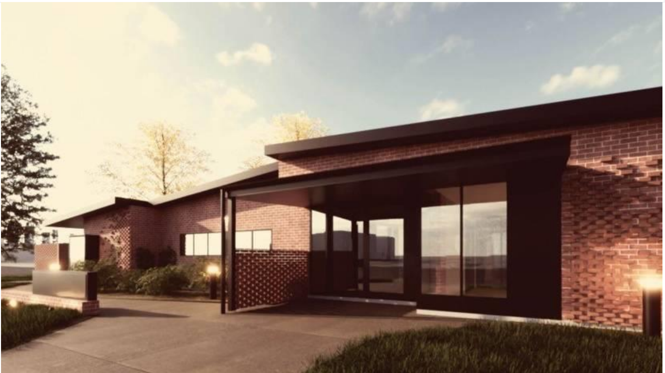
A render of the exterior of Ainslie Group's child care centre. Picture: Supplied
